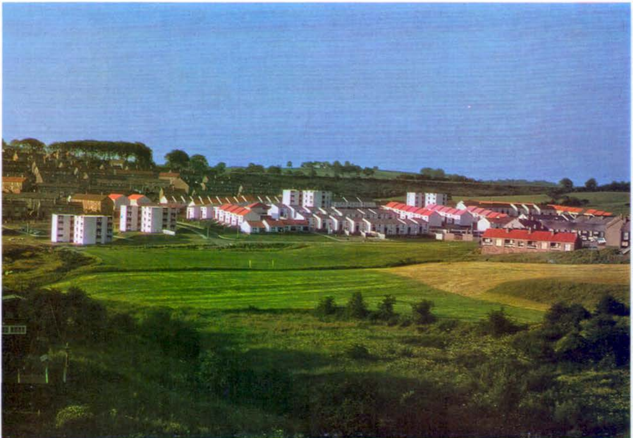
Barshare and Drumdrochan Housing Developments from Glaisnock Viaduct
