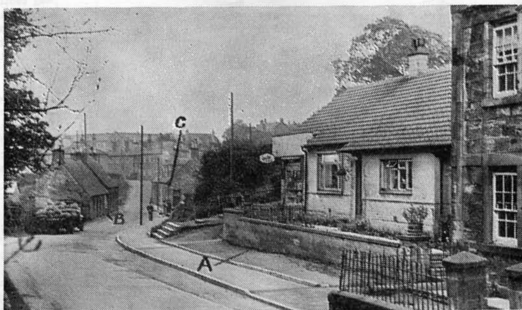
This present-day picture is taken from almost the same angle as the above, the trees on the Townhead Bing making it impossible to get exactly the same shot. The steps indicate the entrance to John Baird Street and Urbana Terrace.
