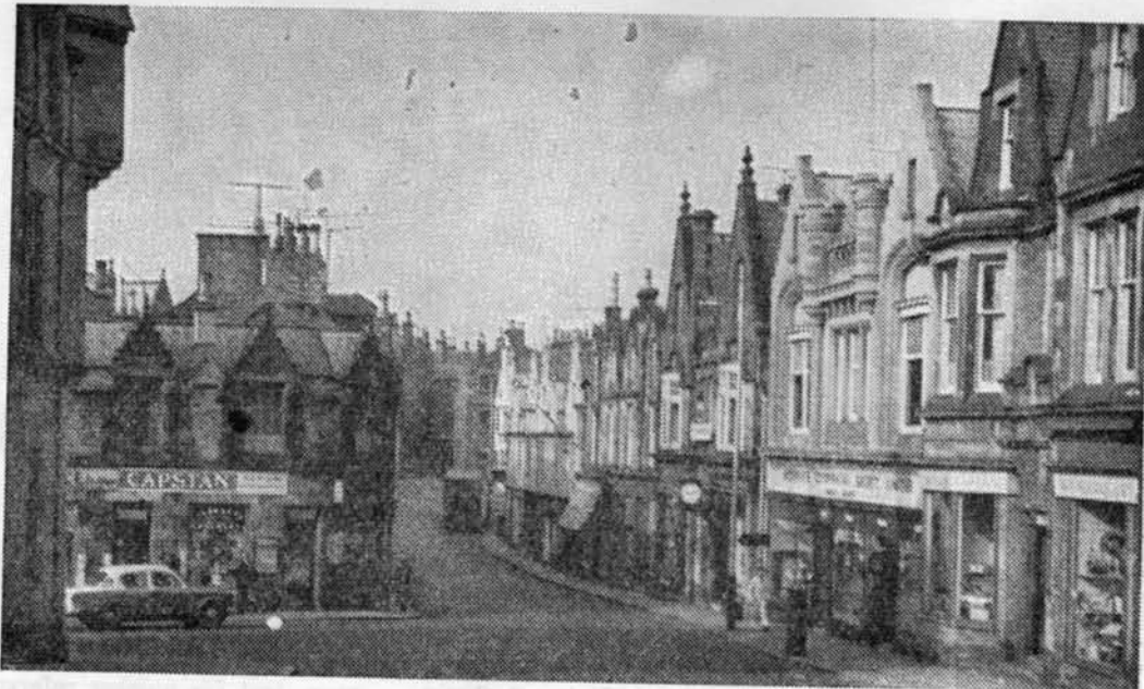
Glaisnock Street and Ayr Road Corner to-day.
