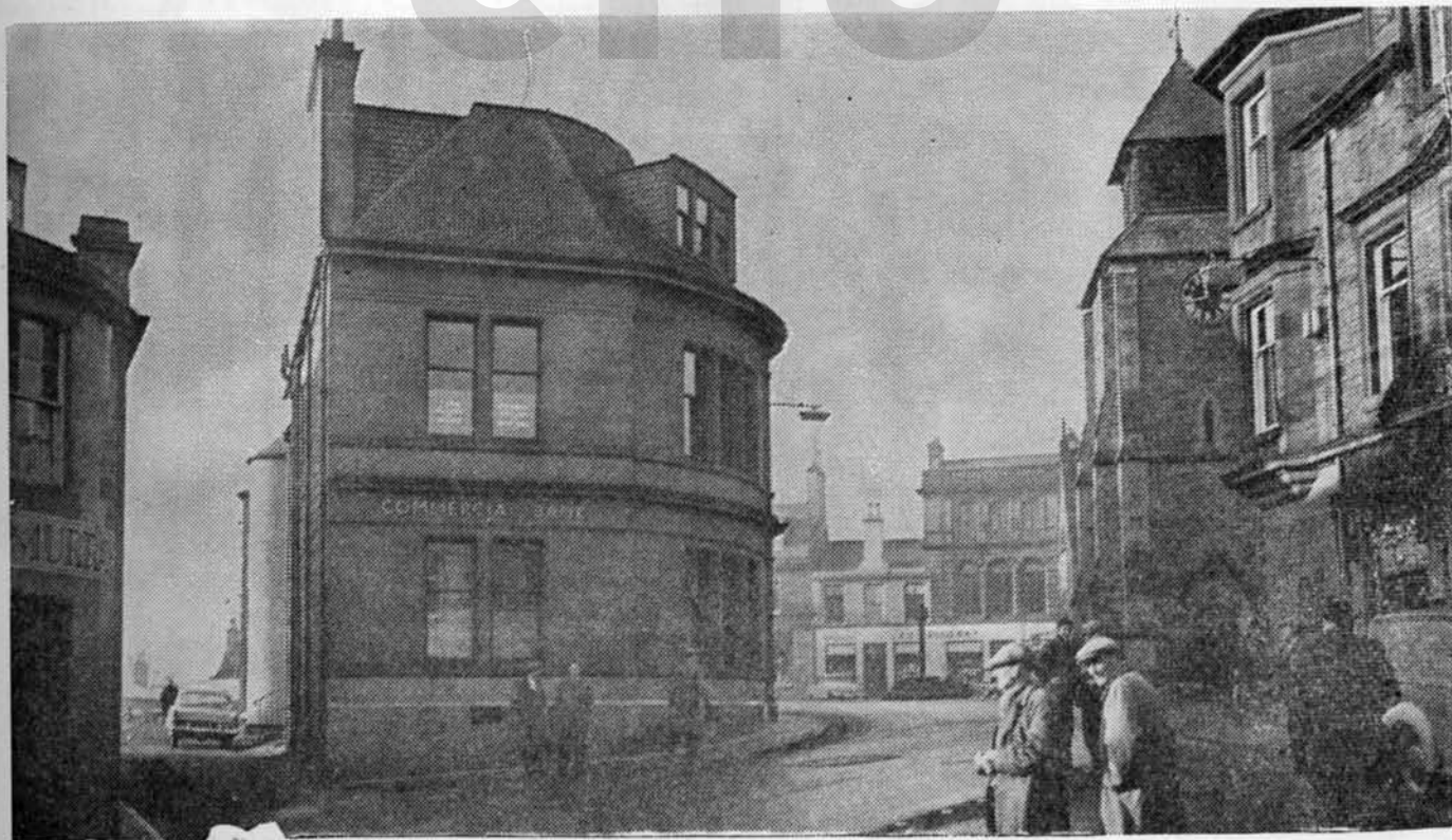
In this fairly recent photograph the roadway is still open from Glaisnock Street to Tower Street. Note how additional main-road width was obtained by curving the bank corner.
