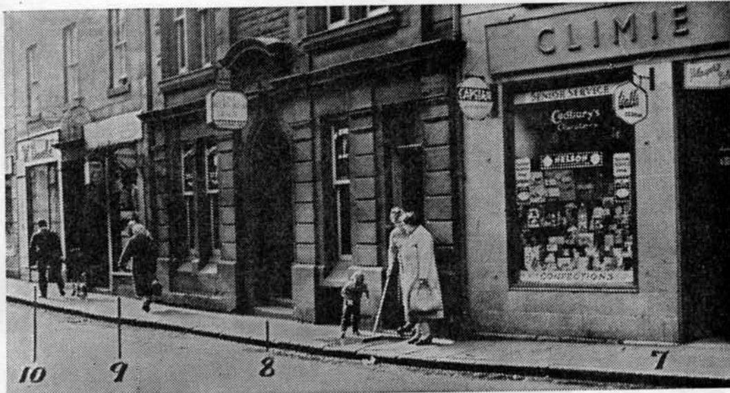
Another section of Glaisnock Street as it is to-day.
